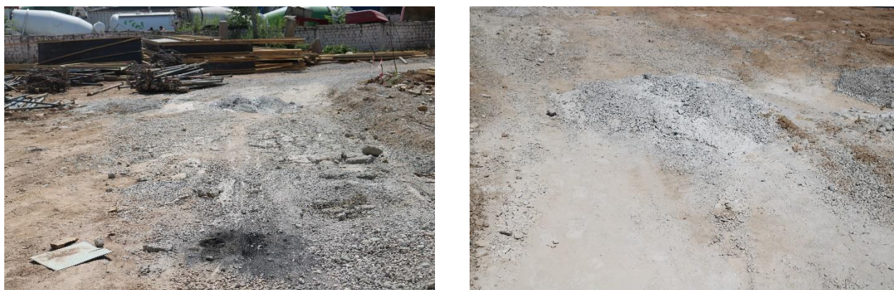
Photo 5: Ingress of concrete mix to the site. May 2023
