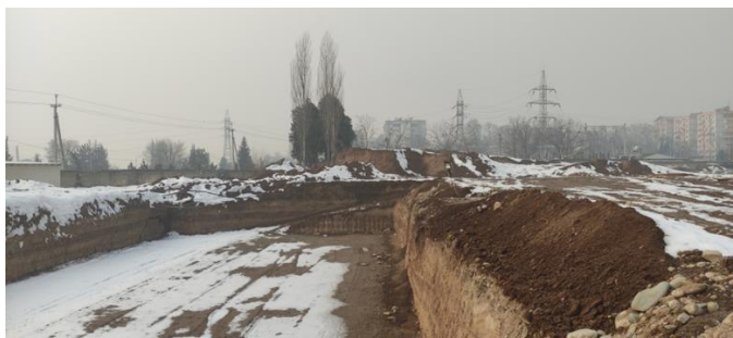
Photo 6: Foundation pit excavated, December 2022
